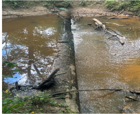
Mill Creek Wastewater Creek Crossing
