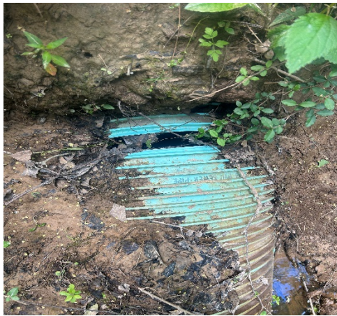
Mill Creek Wastewater Trunk Main
