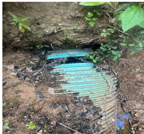
Mill Creek Wastewater Trunk Main
