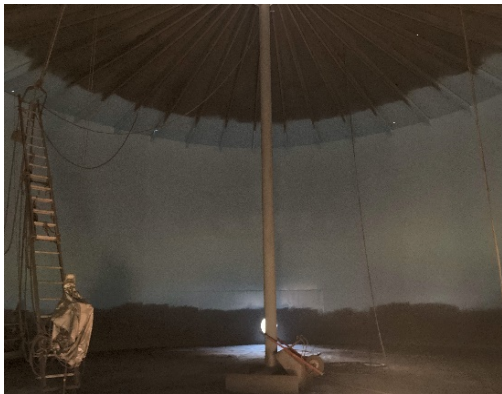
Ragley 1,500,000 Million Gallon Tank
